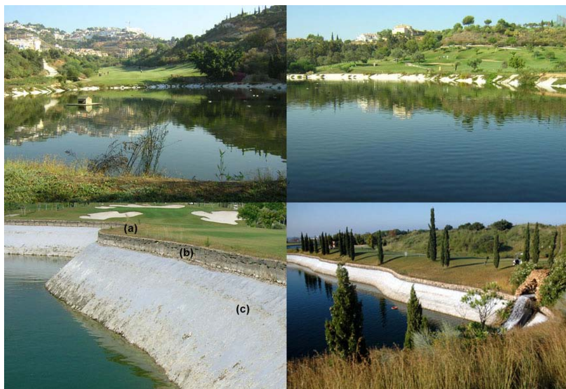
Figure 4. Types of artificial lakes inhabited by otters in golf courses. Details of the artificial lake shores: poor vegetative coverage (a), stone breakwater (b) and roofing felt (c). Photo: Jesús Duarte.
