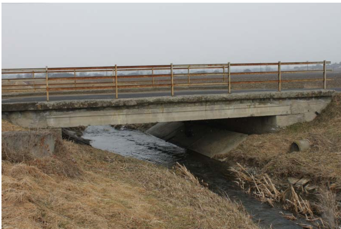
Figure 5. Example of an otter passable bridge in Mučínský potok (brook) (photo P. Urban)
