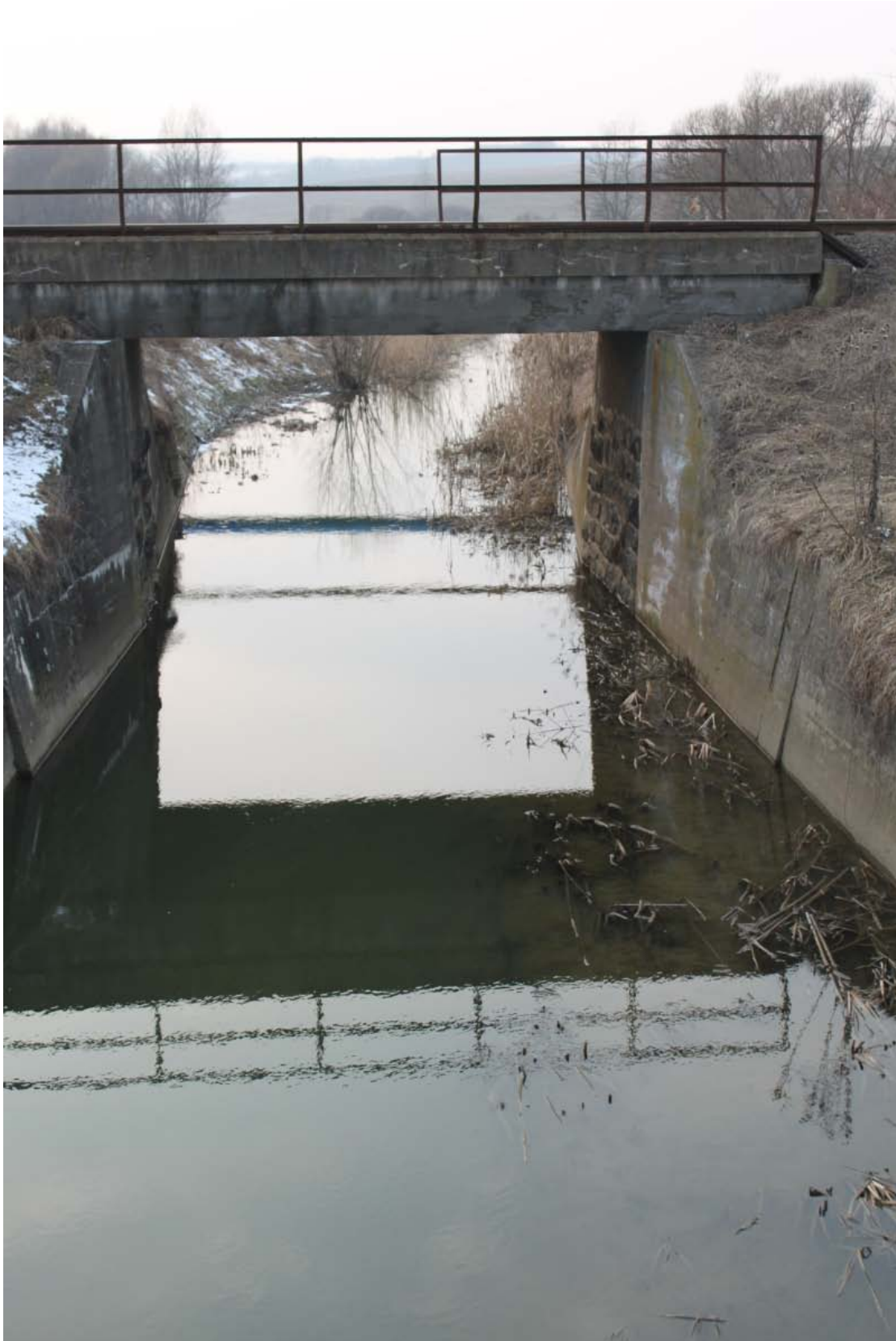
Figure 6. Example of an otter unfriendly bridge in Fekete víz (brook) (photo P. Urban)
