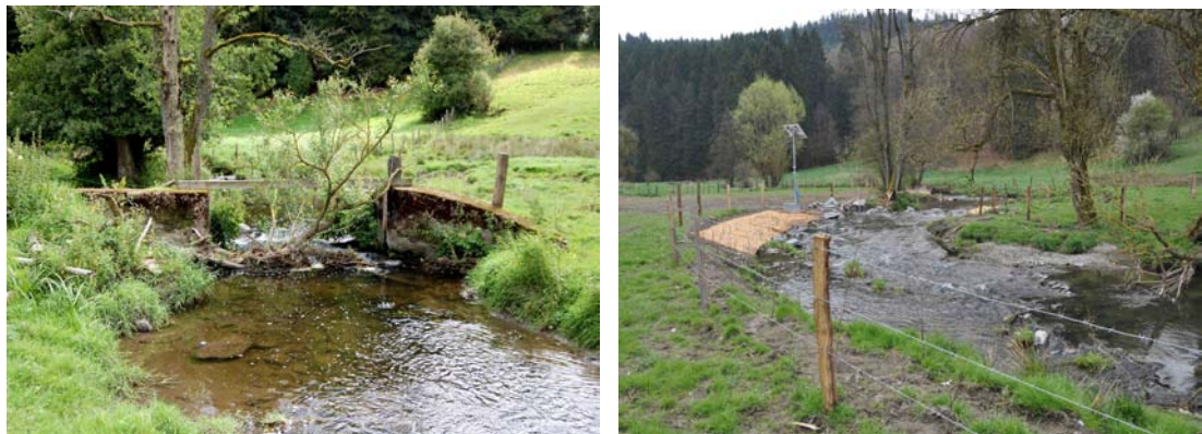
Figure 10. The removal of a concrete obstacle on the Wiltz River (before and after the work).
