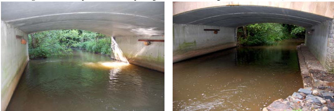
Figure 13. Example of a local stone passage under a bridge along the Wark River (Welscheid) (before and after the work)
