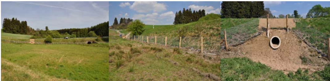
Figure 12. Example of a culvert passage with fences along the Troine River (Neimillen).
