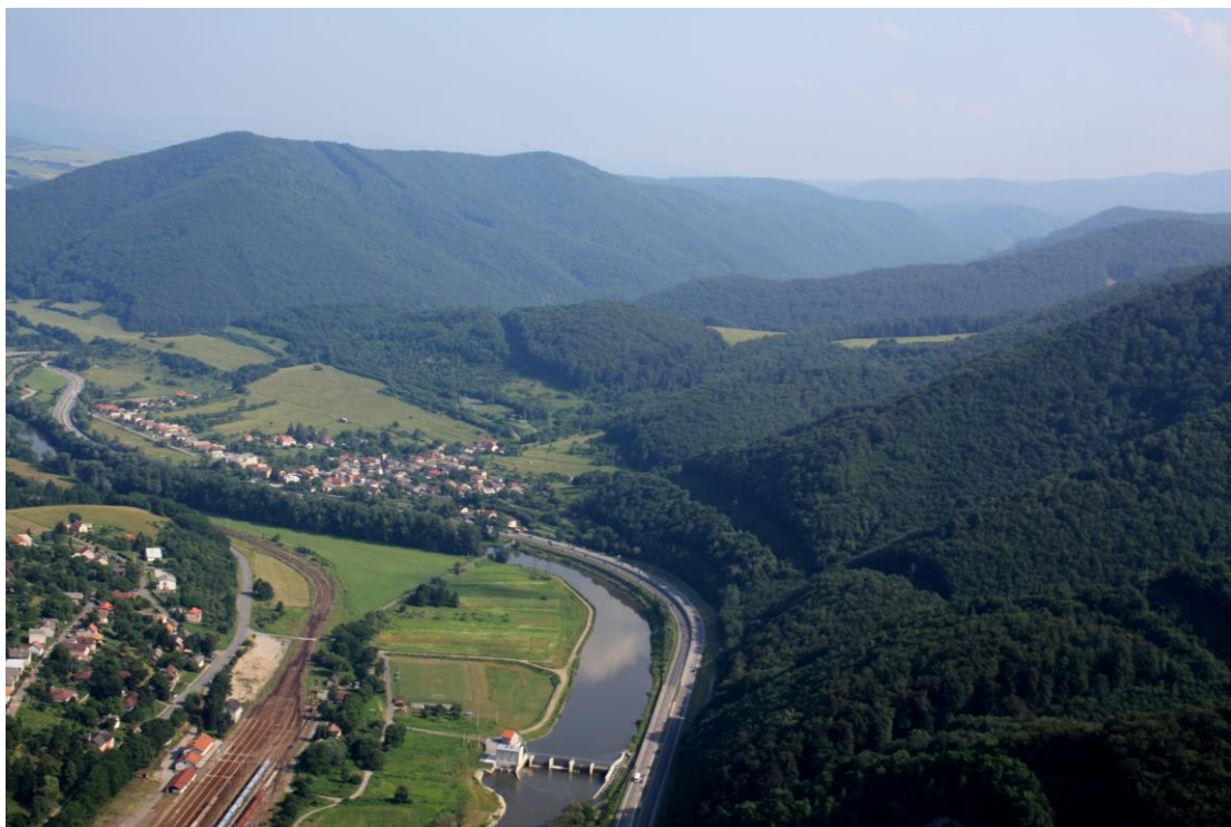
Figure 14. Hronská Dúbrava small hydroelectric power plant was built in 2011 © Peter Urban
